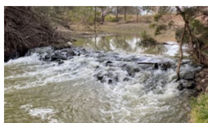
Instream works (block bank)
