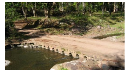
Culvert crossing on a river
